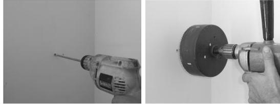
Outside the building, find the pilot hole. Using a hole-saw, with the pilot hole as a guide, drill a 6 1/4" hole.
