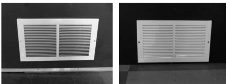
When the flow is limited or inaccessible between rooms downstairs (if there are walls or partitions), then install a grille 8" x 10" (or other grill configuration, having total area of not less than 80 sq. in.) in the bottom of the door or wall to avoid having stagnant air in those areas. Otherwise interior doors must remain open. This insures that all the air drawn into the Humidex comes from all areas of the basement.
